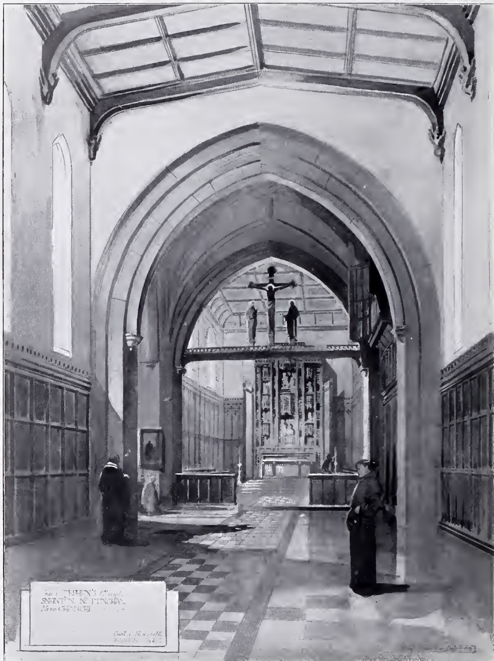
1561. St. Stephen's Church, Sneinton, Nottingham. New Chancel. CECIL G. HARE, Architect. Contractor: R. Bridgeman, Lichford.
